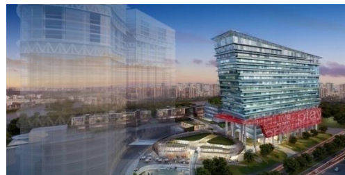
Fusionopolis Phase 5 To Complete in 2014
