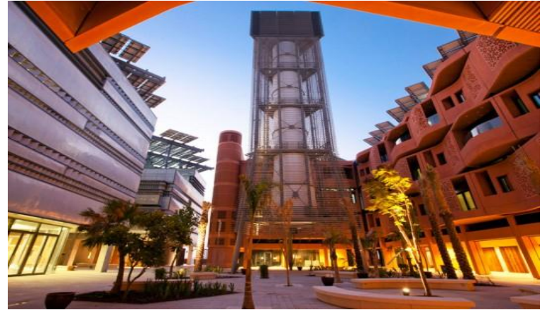
District Cooling, Abu Dhabi
