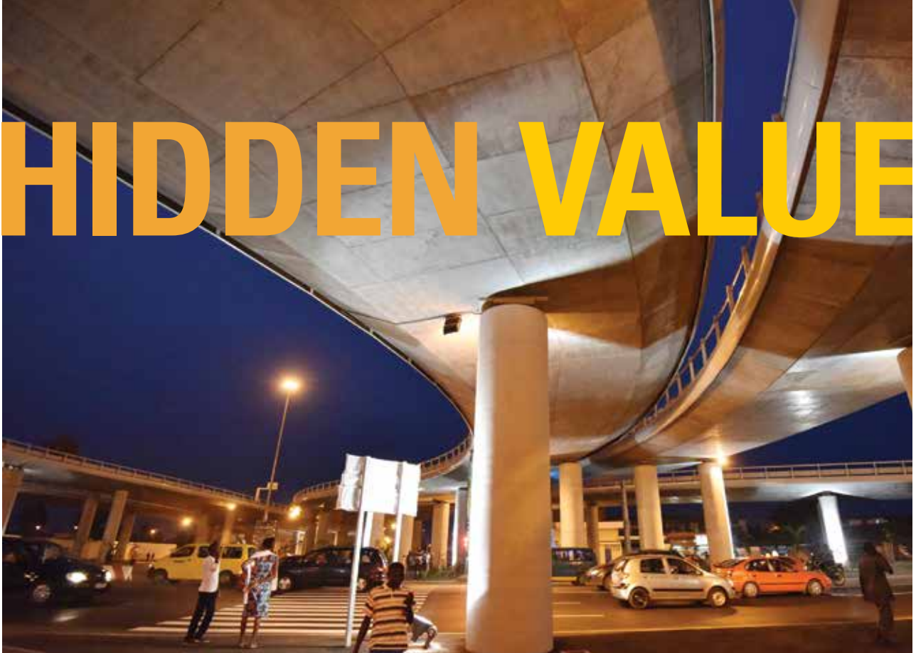
Henri Konan Bédié Bridge, a public-private partnership, links the north and south of Abidjan, Côte d'Ivoire.
