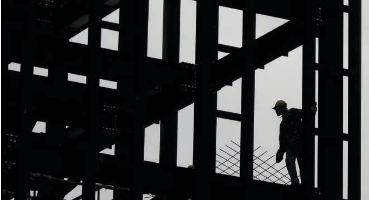
Laborer works on building under construction in Athens, Greece.
