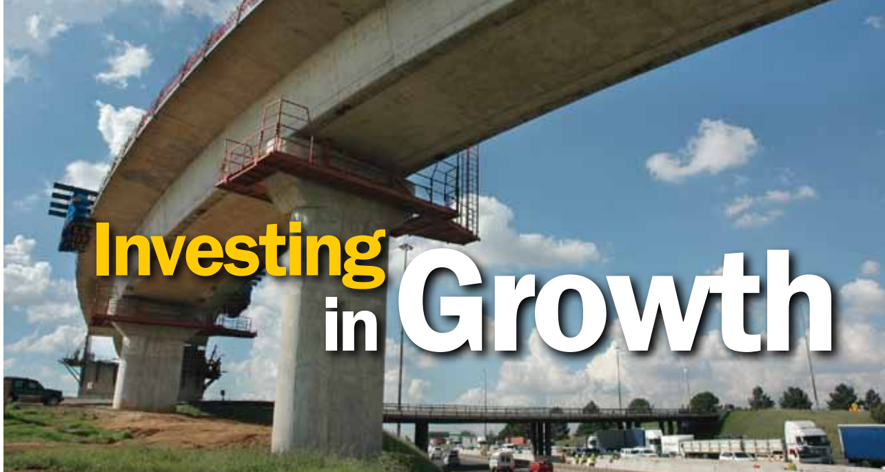
Highway interchange construction in Johannesburg, South Africa.
