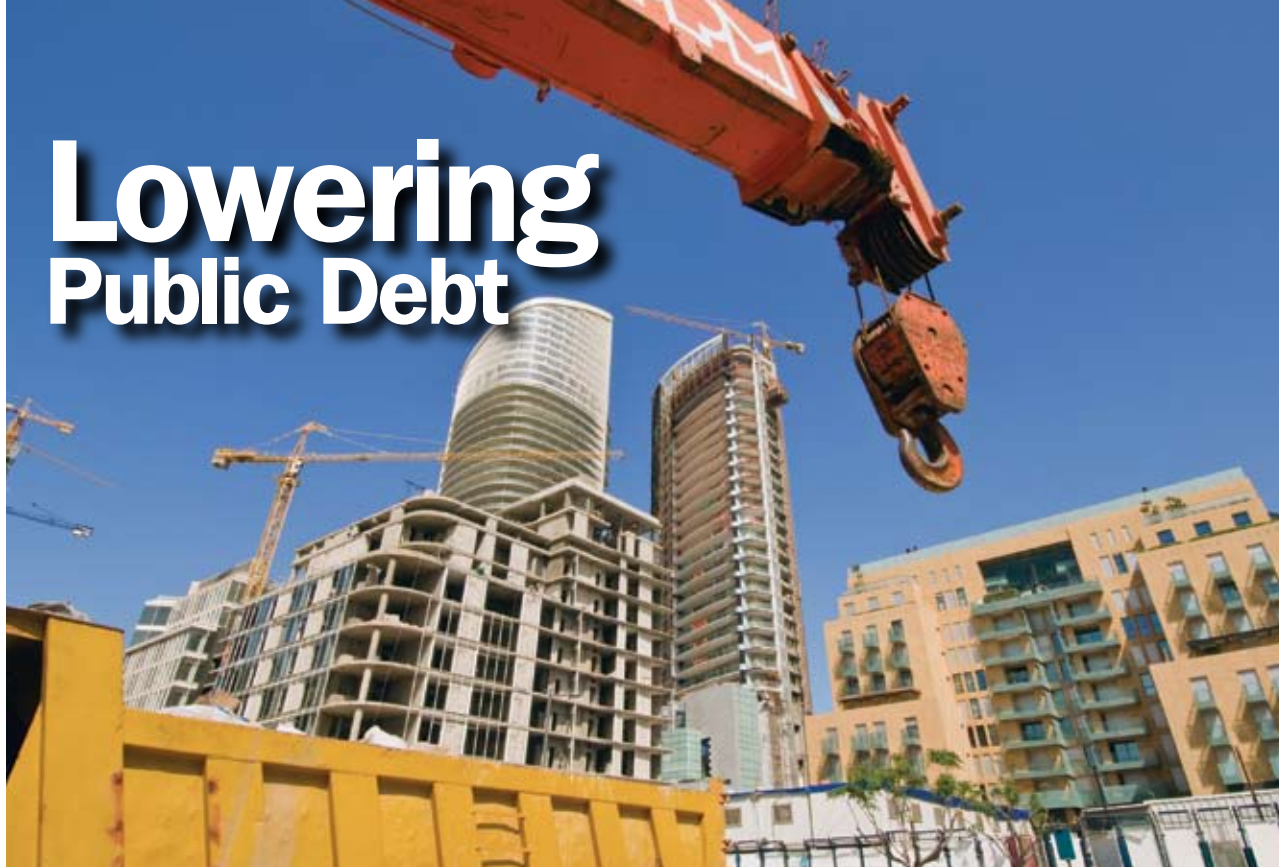
Construction in Beirut.
