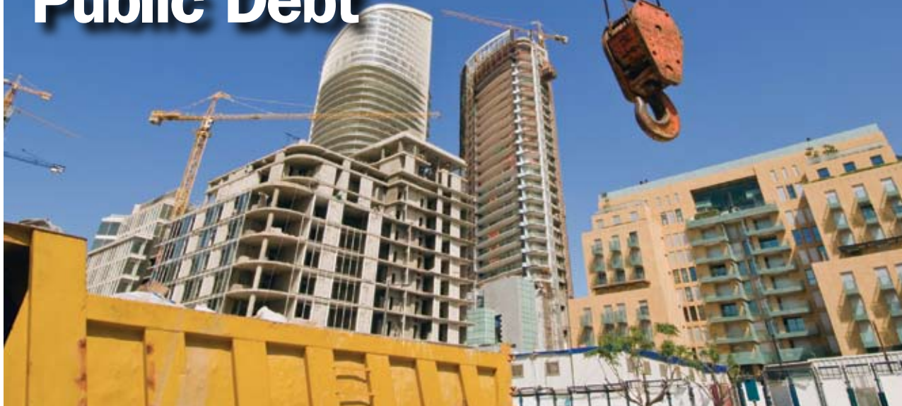
Construction in Beirut.
