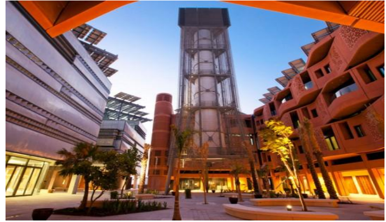
District Cooling, Abu Dhabi
