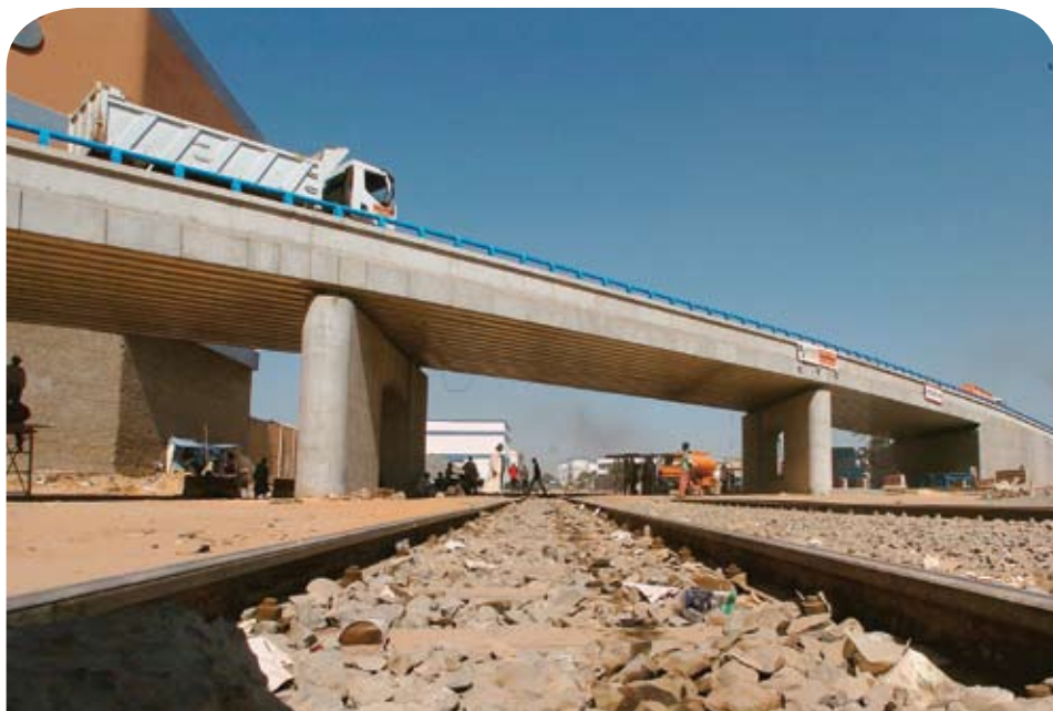
Construction in Dakar, Senegal: IMF–World Bank debt issuance plan includes focus on bond financing for African infrastructure.
