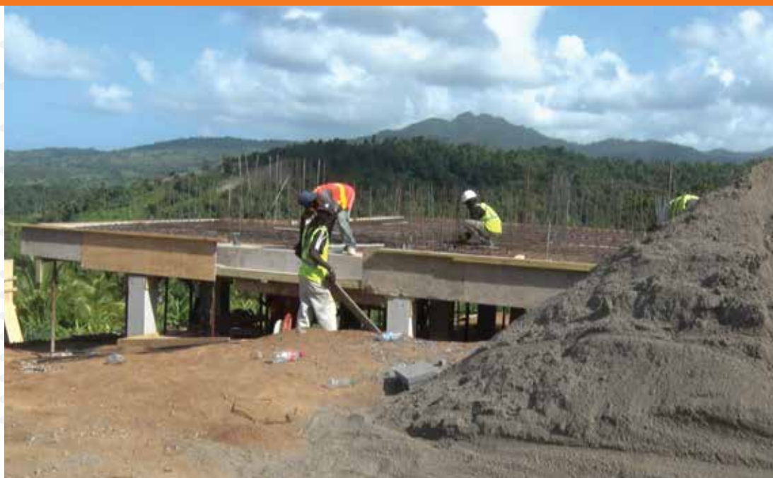
Rebuilding climate-resilient housing and a clinic in Dominica.
